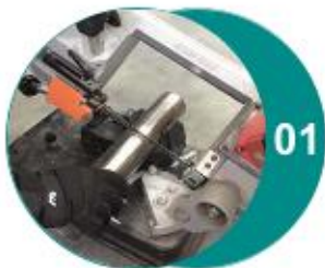
Use cutting machine to cut the pipe.
