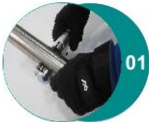
Use pipe cutter to cut the pipe.
