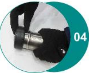
Insert the pipe ends into the seal to 2-3 cm on each side.
