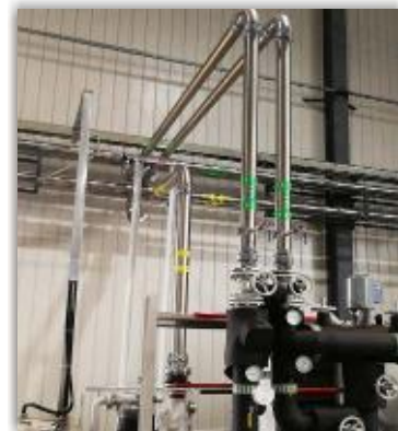
● Oil and Cooling water for Machinery.
