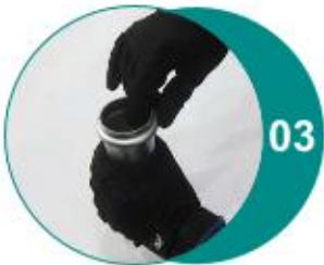
Visually check the seal is seated.
